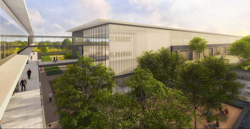
COLLIN COLLEGE TECHNOLOGY CAMPUS 340,000 SQUARE FEET OF CLASSROOM, LAB AND OFFICE SPACE
